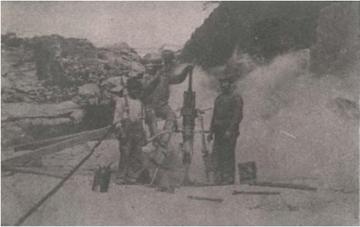
Steam drills and operators.
